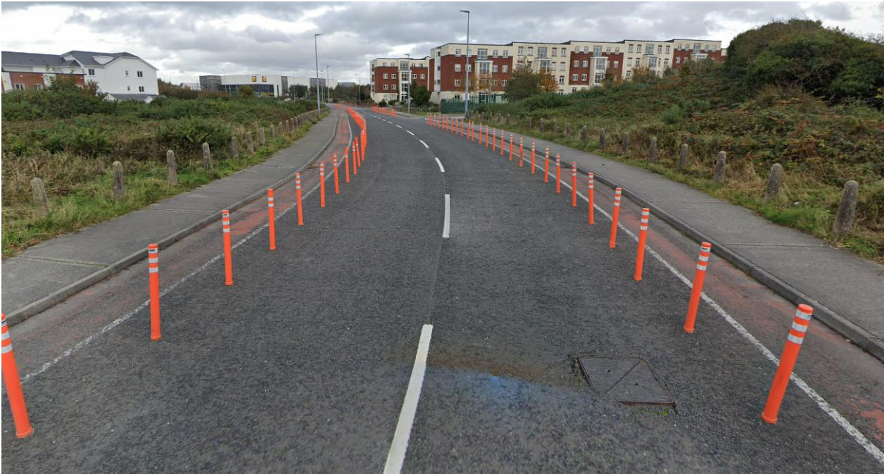
Figure 3- 7: School Access Road (Looking North) (Ref: https://www.google.ie/maps )
